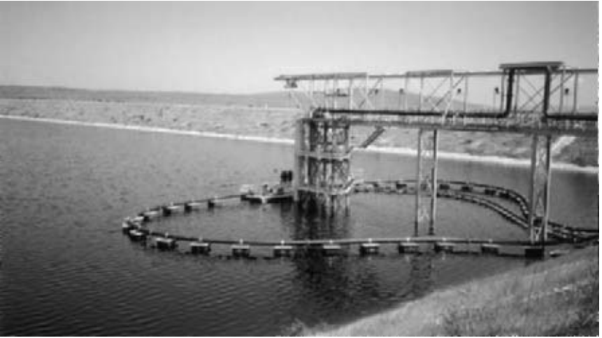
FIGURE 6 Float-mounted pumps designed to skim the clean liquid in a settling pond (Hazleton Pumps, Inc.)
