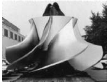
FIGURE 4 Mixed flow propeller runner (Voith Siemens Hydro)
