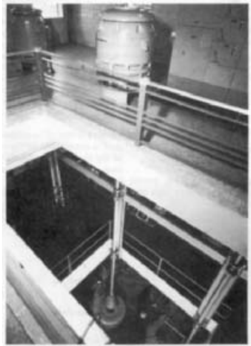
FIGURE 22 Sections of flexible shafts and intermediate guide bearings used to transmit torque from motor located above flood elevation to pump located below ground (Flowserve Corporation)
